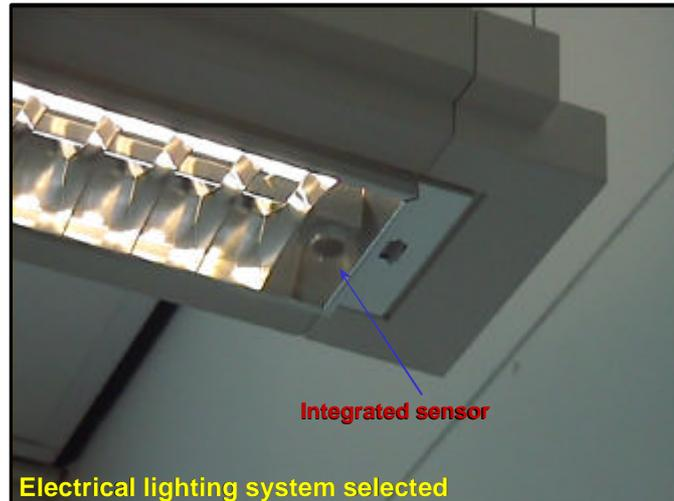
Figure 62: Electrical lighting system with integrated sensor and control.
